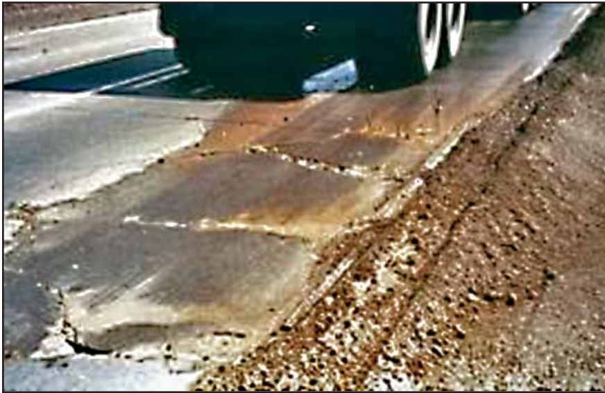
Third-stage cracking and pumping.
