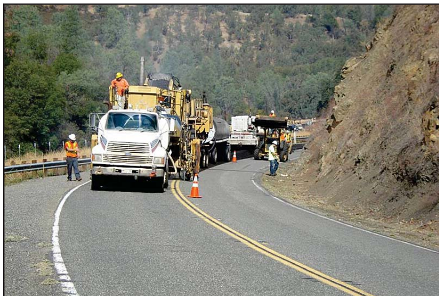
Picture 1. Surface recycling operations near Williams, Calif.
