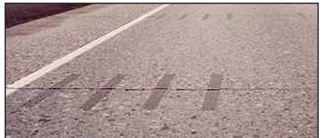
Above, dowel bar retrofit of fatigue crack, and below, the completed retrofit.
