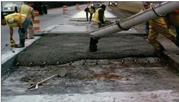
Slab repair will be one topic in the workshop to be presented at the concrete pavements conference. The photo above shows a typical RSC slab replacement.
