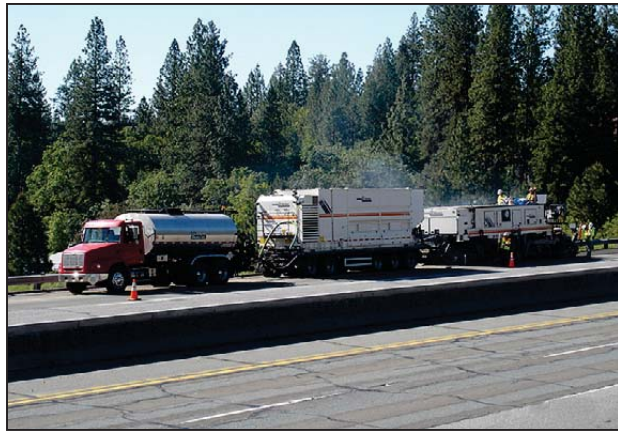
Picture 4. In-place recycle train on I-80 near Auburn, Calif.
