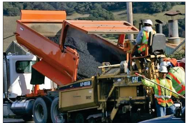
Warm mix asphalt is unloaded at a job site. Photo: Graniterock.
