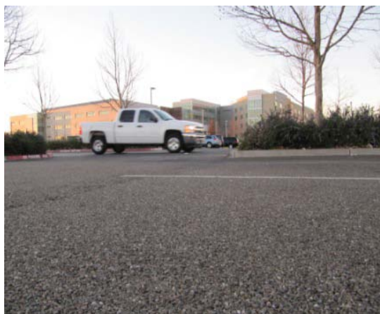
The porous asphalt parking lot at Kaiser in Modesto
