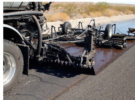
Application of PASS CR for the scrub seal
