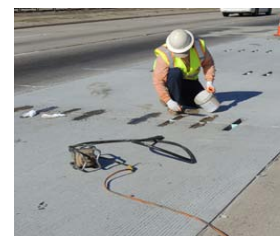
Dowel bar installation was performed the following shift
