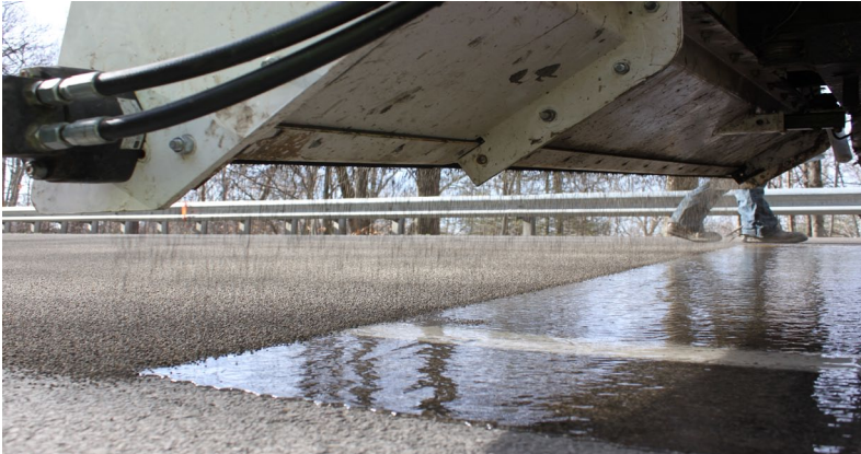
HFST aggregate application
