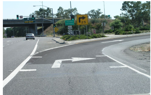
HFST on an off-ramp
