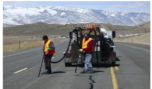
Crack sealing in cool weather
