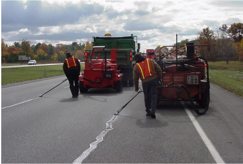
Sealant material being injected into cracks on highway
