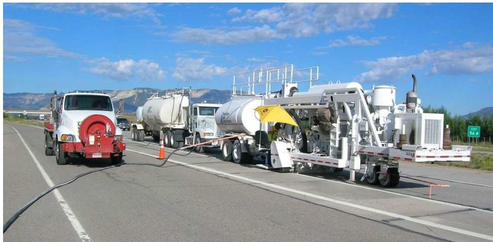
Diamond Grinding Operation
