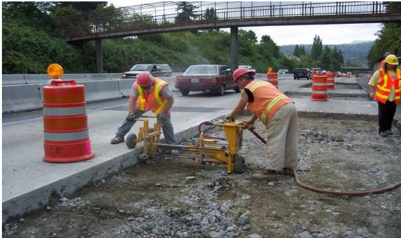
**Figure 5. Drilling holes for tie bars.**
