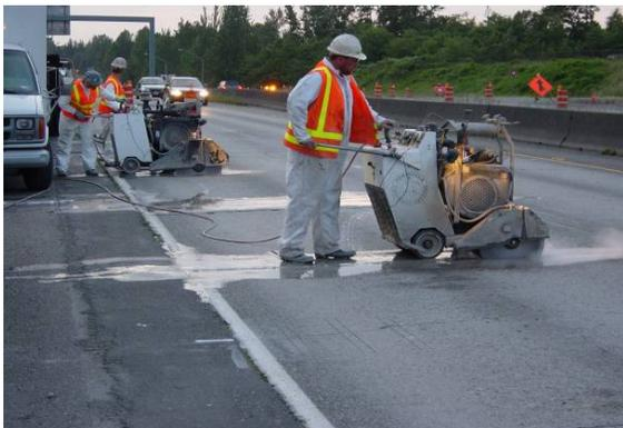
**Figure 1. Perimeter sawcutting.**
