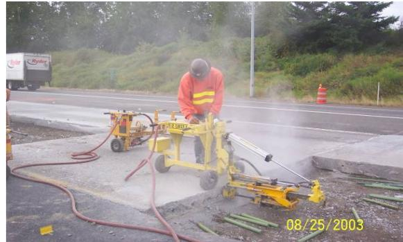
**Figure 6. Drilling holes for dowel bars.**
