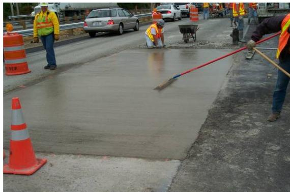
**Figure 9. Finishing concrete.**
