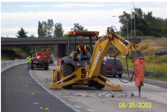
**Figure 3. Removal with backhoe hoe point**
