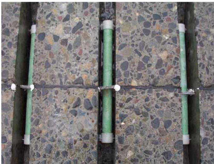
**Figure 5. Dowel bar retrofits at a transverse joint (8).**
