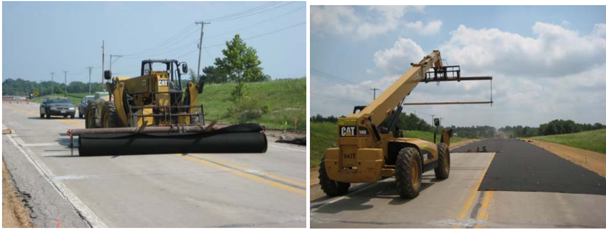
Figure 6. Geotextile fabric placement.
