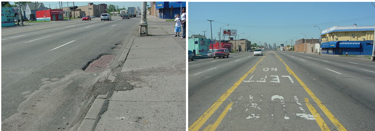
Figure 8. Condition of existing composite pavement.
