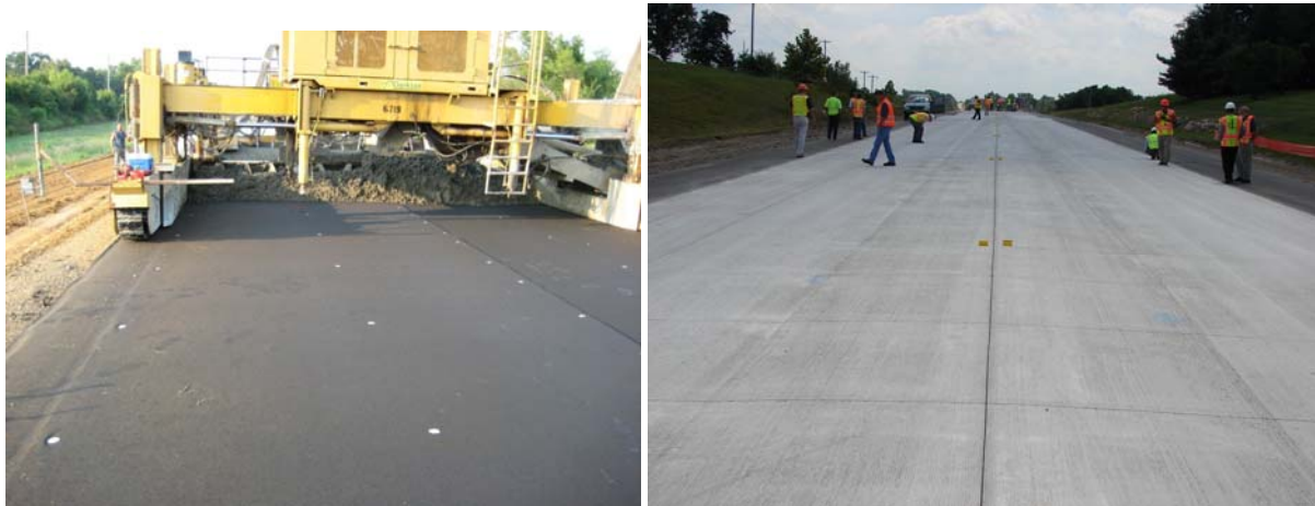
Figure 7. Slipform paver over the fabric and completed unbonded overlay.
