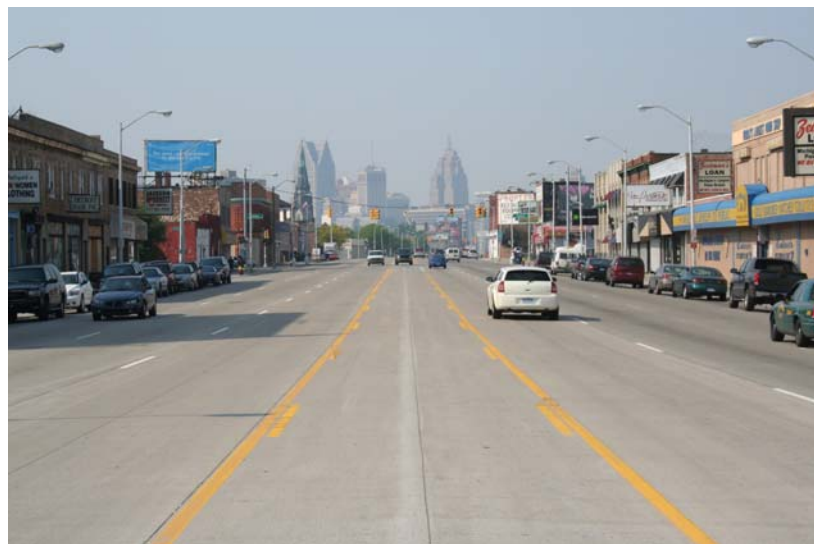
Figure 11. Completed thin unbonded overlay.
