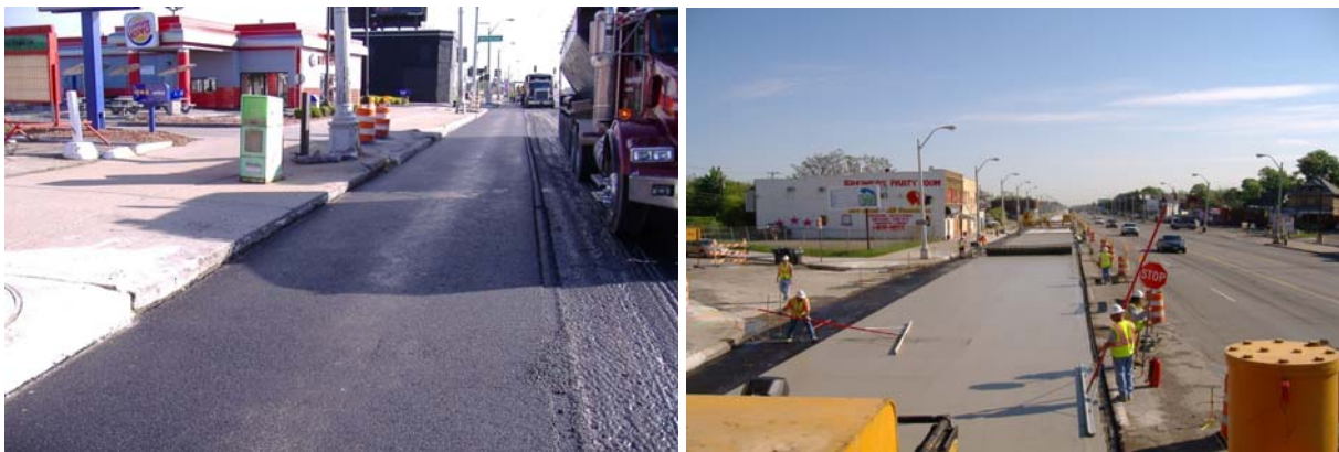
Figure 10. AC interlayer and concrete placement.
