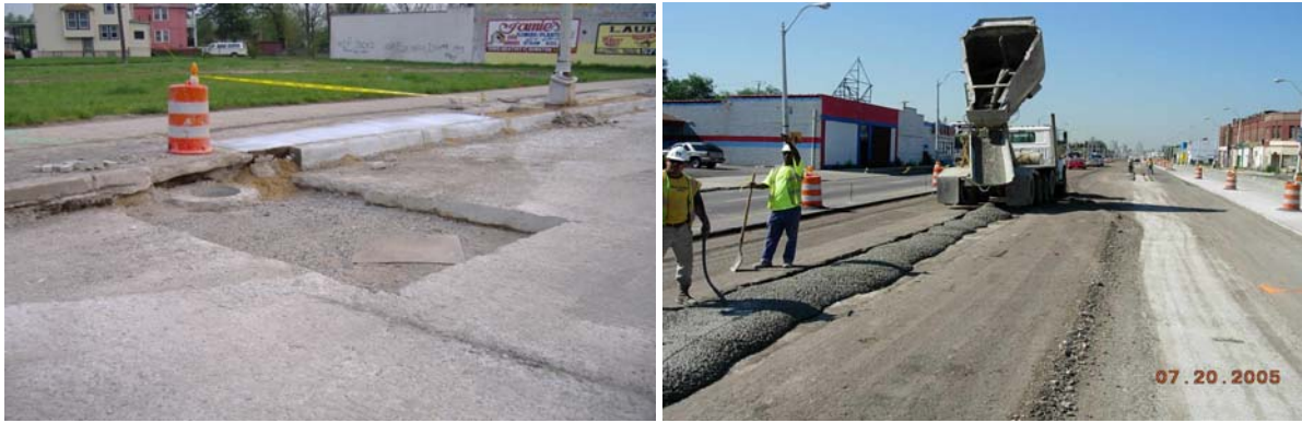
Figure 9. Pre-overlay repairs.
