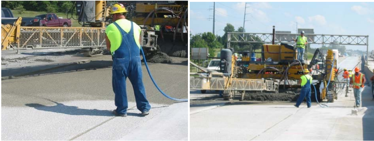
Figure 4. Slurry application and concrete placement.
