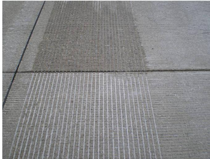
**Figure 11. Longitudinal grooving completed perpendicular to the transverse tines.**
