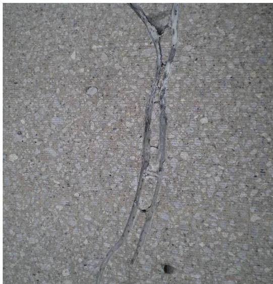
**Figure 5. Cracking at a stitch that was completed too late.**
