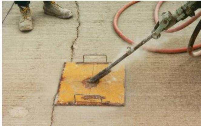
**Figure 2. Drilling holes for cross stitching.**
