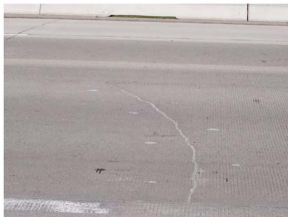
**Figure 4. Completed crack stitch.**
