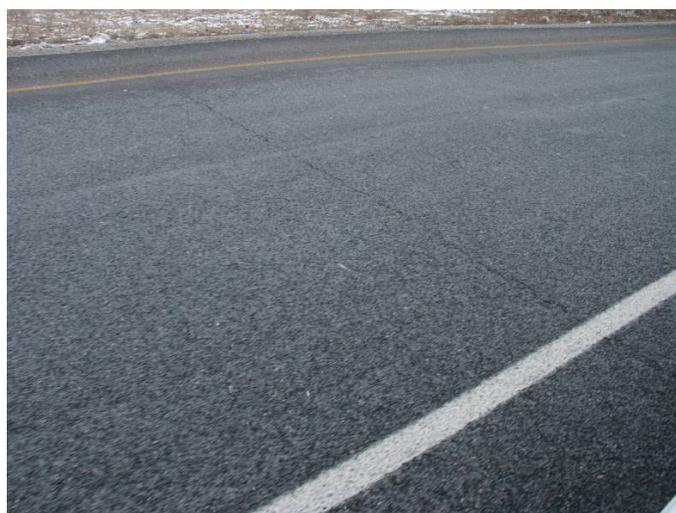
**Figure 19. Thin asphalt concrete overlay over a concrete pavement.**
