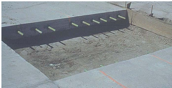
**Figure 15. A 2-m full-depth repair area prepared for concrete placement.**
