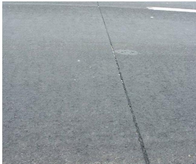
**Figure 18. Micro-surfacing over a concrete pavement.**
