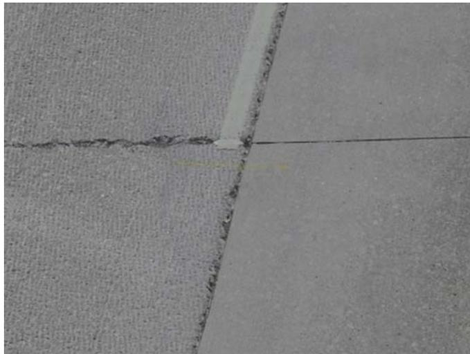
**Figure 10. Difference between micro-milling (left) and diamond grinding (right).**
