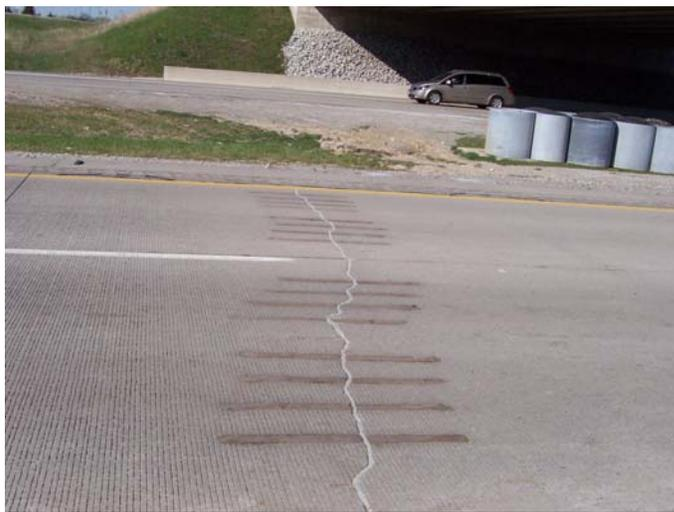
**Figure 8. Load transfer retrofit for a mid-panel transverse crack.**
