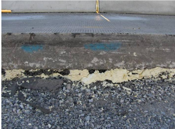
**Figure 14. Slab jacking using foam.**
