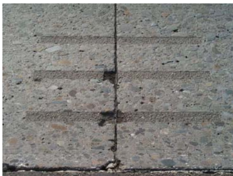
c. Spalling
