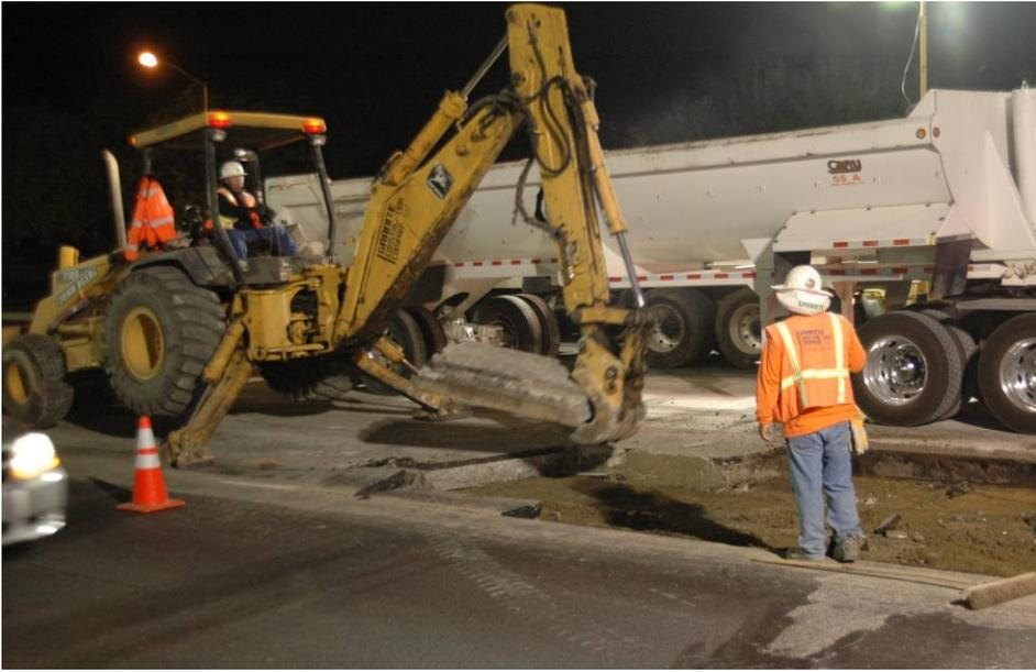
**Figure 2. Damaged highway panel being removed.**
