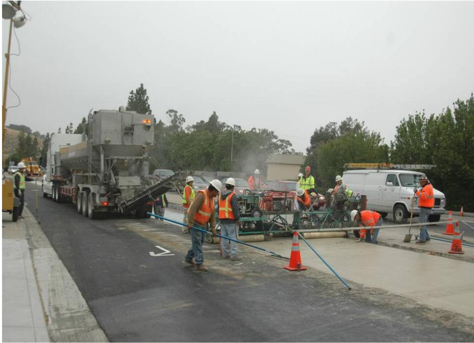
**Figure 4. Finishing the panel.**
