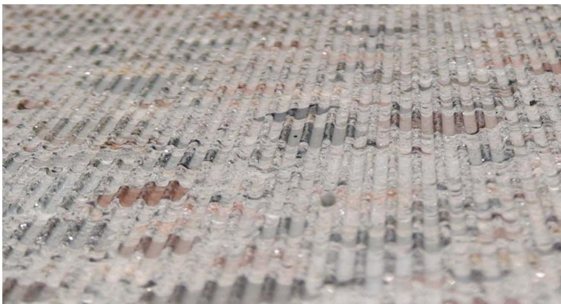
**Figure 12. MnROAD I-94 conventional diamond-ground texture after 5 months of traffic.**
