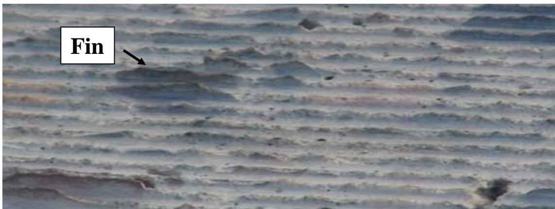
**Figure 3. Variability of fin profile on conventional diamond-ground surface on MnROAD I-94.**
