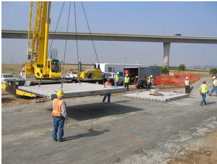
**Figure 3. The construction the HVS testing-site for the precast pavement rehabilitation for the I-15 Ontario project.**
