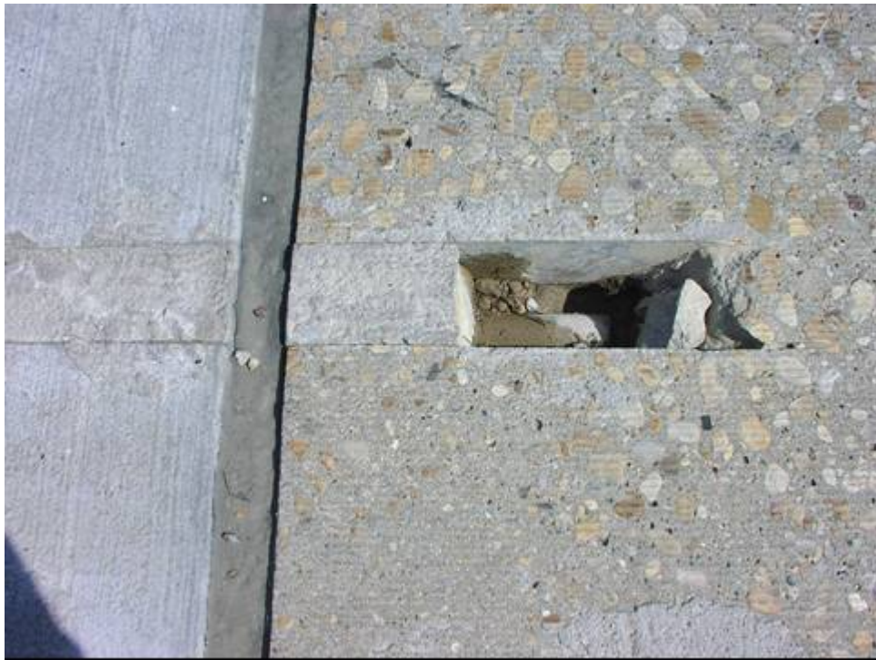
Figure 3. Exposed dowel.
