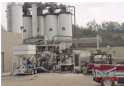
CRM is blended with hot asphalt cement
