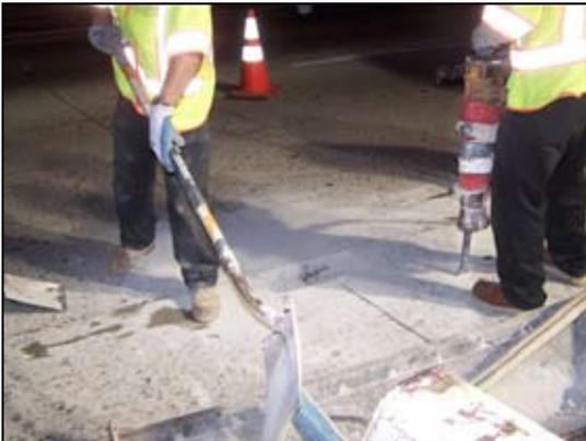
that does not fully extend through a concrete slab. This method is used to repair spalling and fraying of concrete slab edges at joints and cracks as well as localized scaling. Spalling, which can occur on both jointed and continuously reinforced pavements, reduces pavement serviceability and can become hazardous to highway users. This type of deterioration can be caused by a
