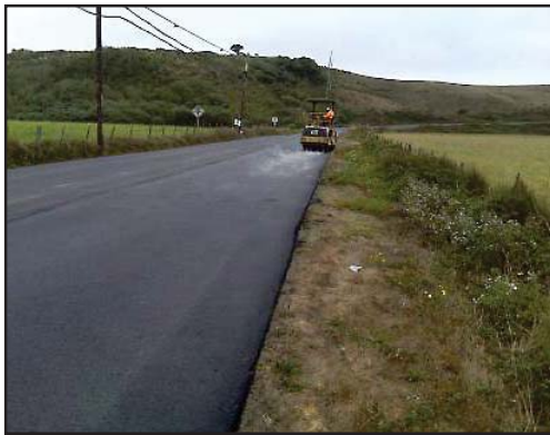
Figure 2: Compaction.
