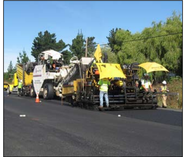
Paving train; note lack of smoke.
