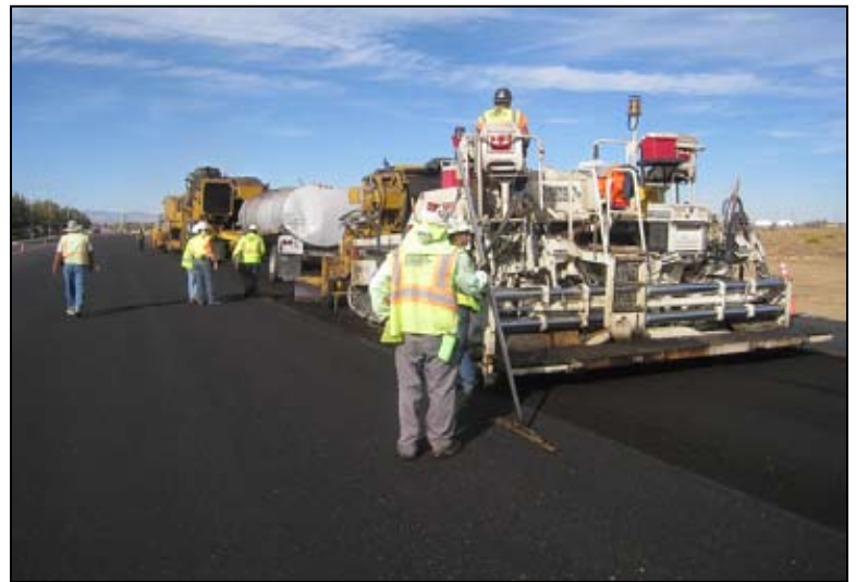
60th Street west during construction of last lane of CIR.
