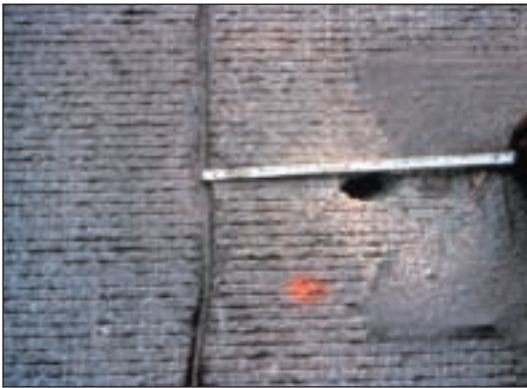
3. Checking hole location.
