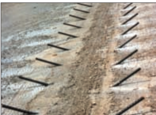
5. Inserting bars into prepared holes containing epoxy. (Note: The bars shown here are in position but not fully inserted.)
