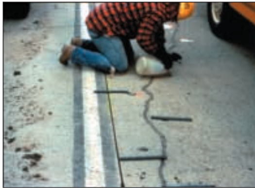
4. Pouring epoxy into drilled holes. (Injecting epoxy is preferable for large quantities.)
