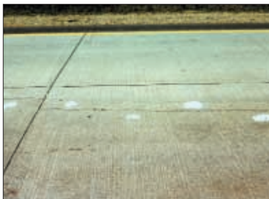
6. Completed cross-stitching on longitudinal crack.
