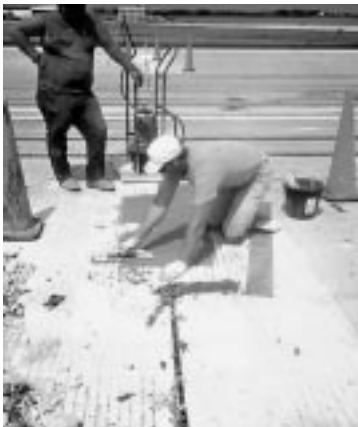
Figure 13.3. Finishing the patch surface.
