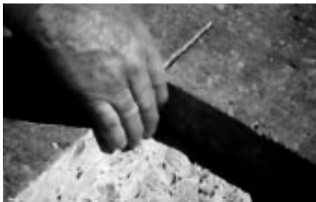
Figure 9.5. Checking for dust & debris within spall repair area.
