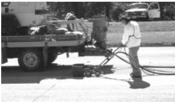
Figure 7.2. Sandblasting a joint face.
