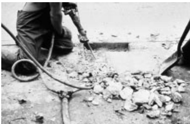
Figure 11.2. Using a jackhammer to remove damaged concrete.
