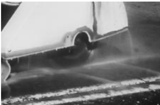
Figure 11.1. Sawing out the edges of a spalled area.
