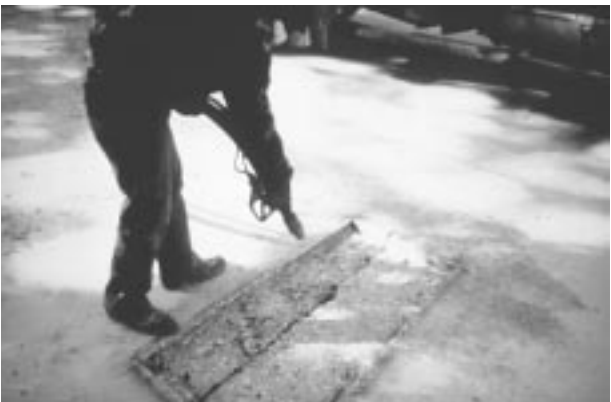
Figure 9.4. Air-blasting to remove dust and debris.
