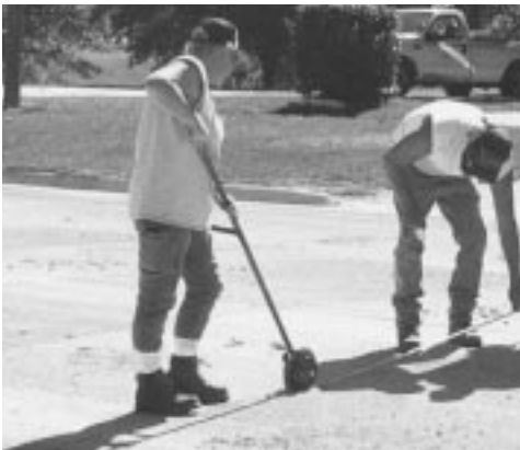
Figure 6.6. Installation of backer rod.
