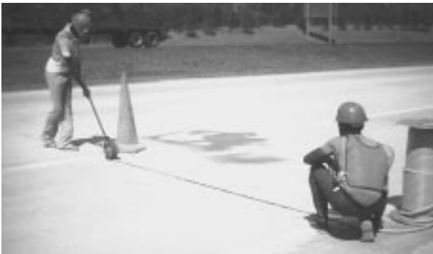
Figure 4.1. Installation of backer rod into joint.
