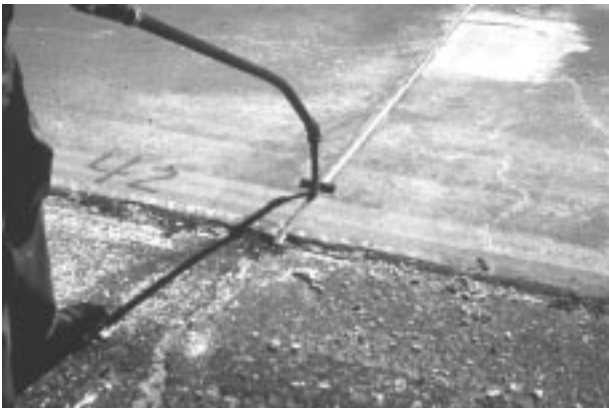
Figure 13.5. Resealing joints after partial-depth repairs complete.
