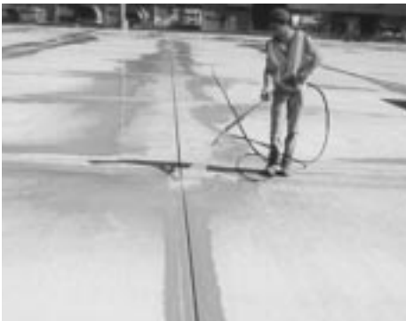
Figure 6.4. High-pressure water cleaning.
