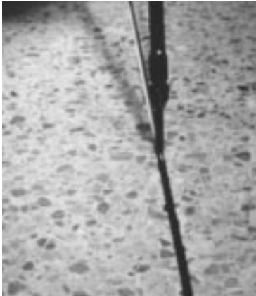
Figure 8.1. Sealing a crack.
