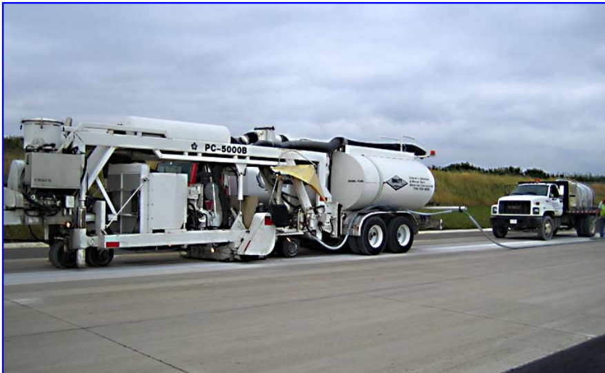
Figure 3. Diamond grinding equipment
