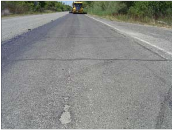
Pavement surfaces can vary just from age and required maintenance.
