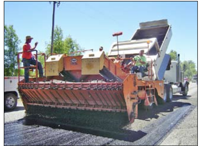
Surface preservation can have many different forms. This is a 'scrub seal' being placed by county crews.
