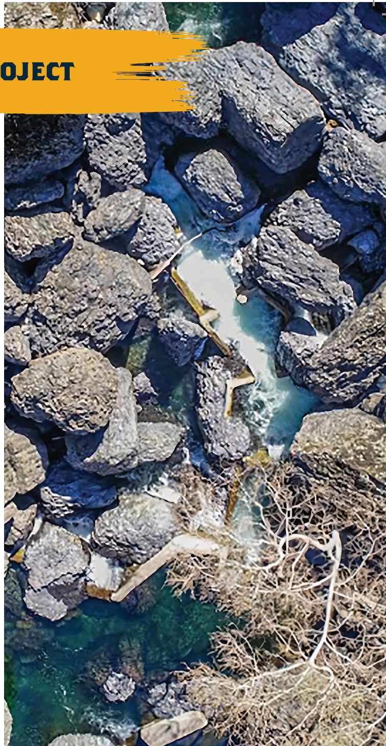
A few of the 70-year-old concrete fish ladder weir that are no longer functional.
