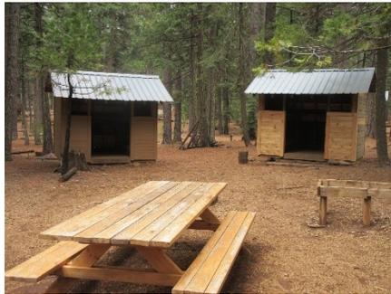
The project for Boy Scouts Camp Lassen consisted of repairing and upgrading 55 Adirondacks buildings that contained 4 beds each. The consisted of removing and replacing damaged siding, re-leveling the units, installing front shear panels, replace the bunk bed plywood and adding 1x trims at the corners and entries. To date, 28 of the 55 cabins have been restored.
