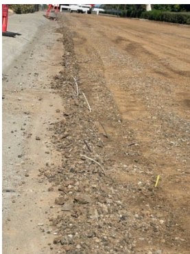
Damaged shallow fiber-optic conduit
