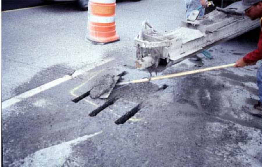
Figure 6-13 Placing backfill (Caltrans, 2006a)
