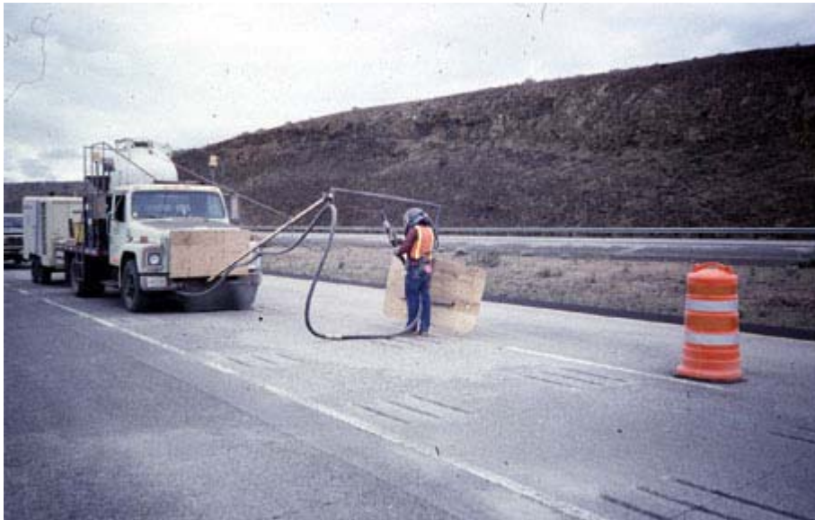
Figure 6-10 Sandblasting (Caltrans, 2006a)
