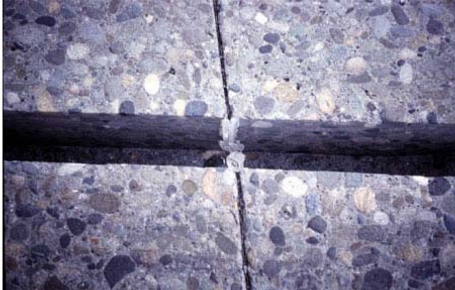
Figure 6-11 Sealing joint/crack (Caltrans, 2006a)
