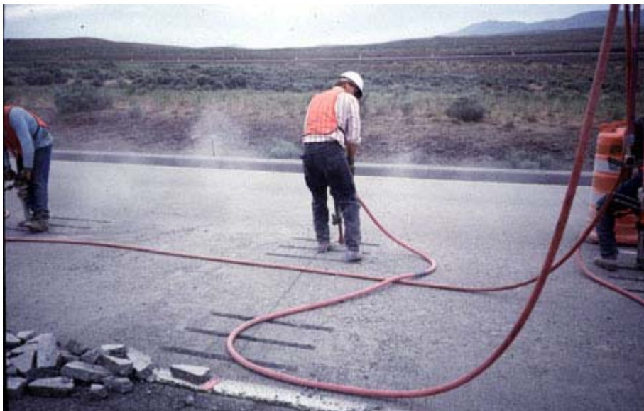
Figure 6-9 Jack hammering (Caltrans, 2006a)
