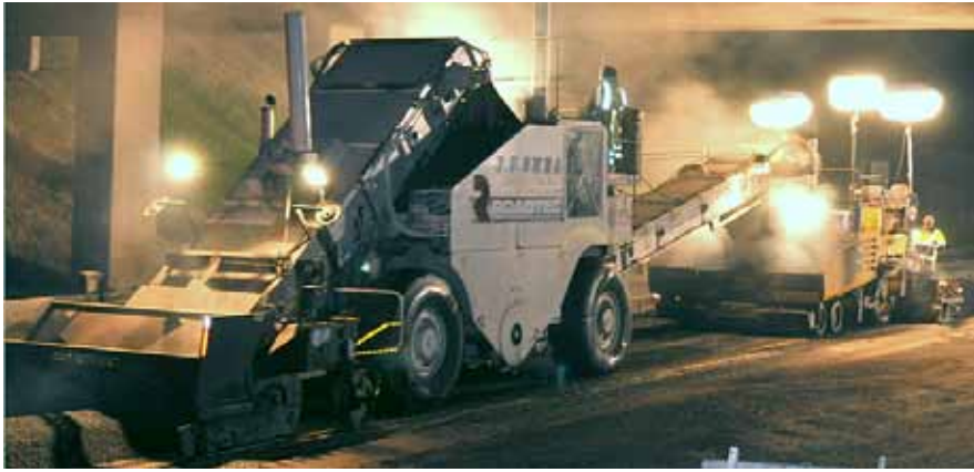
WMA with Evotherm aids cold weather paving on I-5
