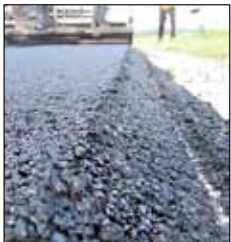
Figure 1. Safety Edge on HMA pavement
