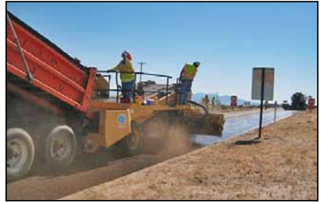
RAP scrub seal being applied on I-10
