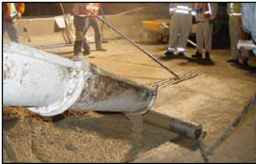
Figure 2. Constructing the replacement slab with rapid strength concrete (RSC).
