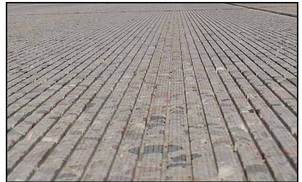
Figure 1. Ground level view of NGCS surface
