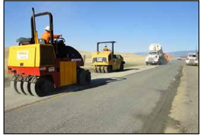
Rolling the chip seal
