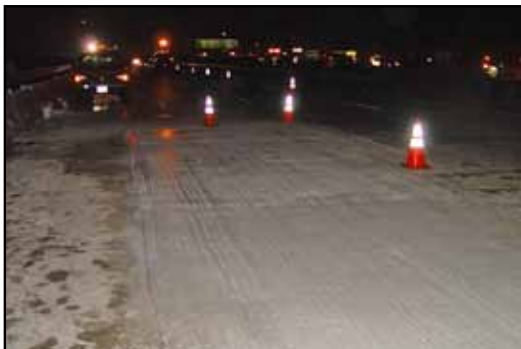
Figure 3. Completed slab replacement with final texture and curing compound.
