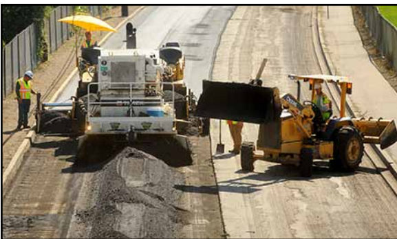
The closed-circuit asphalt recycling plant
