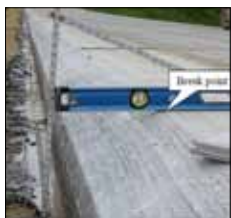
Figure 2. Safety Edge on PCC pavement
