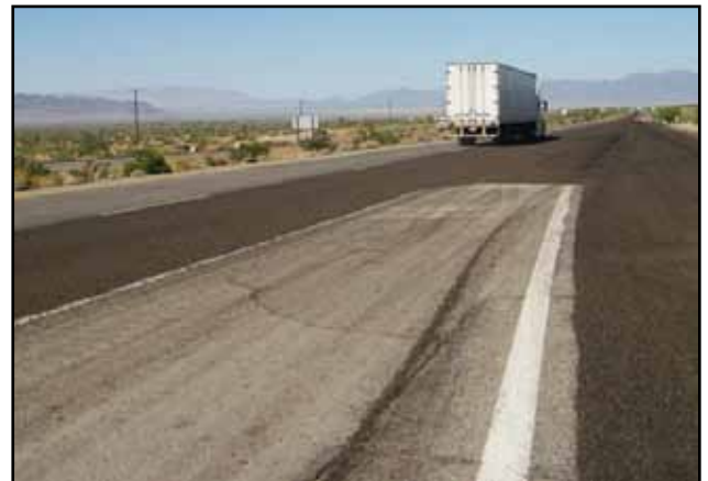
Caltrans' scrub seal application using RAP on I-10
