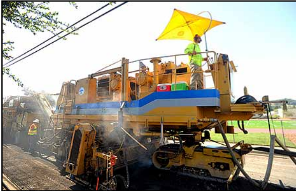
The full-lane 12.5 foot asphalt milling machine
