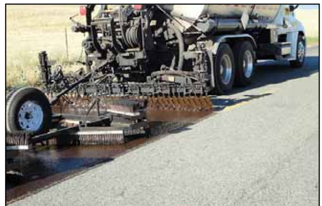
Application of PMRE scrub seal as binder for chips
