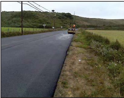
Figure 2: Compaction.
