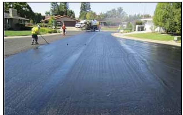
Figure 1 warm mix AR seal coat in construction
