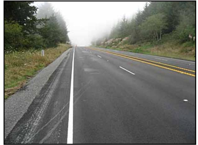
Figure 6 Finished paving with striping
