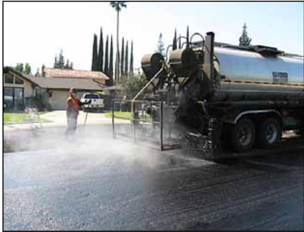
the binder was applied at a rate of 0.25 gal/yd<sup>2</sup> and the chips were applied at a rate of 9-10 lbs/ yd<sup>2</sup>. The warm mix asphalt rubber binder was applied at a temperature of 335 to 340°F, which is a 60°F reduction from the normal application temperature of asphalt rubber chip seals. The temperature reduction lessens the energy used in the heating process, and also reduces the emissions (see Figure 2).
