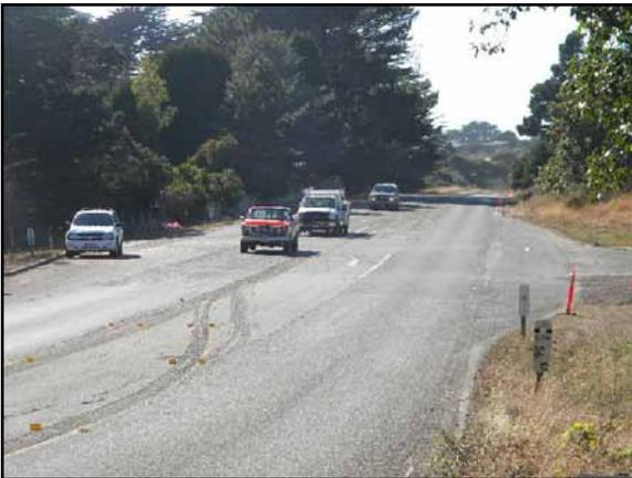
District 4 selected this stretch of road to be built with a Polymer Modified Gap-Graded HMA mixture at a target lift thickness of  $\frac{3}{4}$  inch. The average production was 1,115 tons per day.
