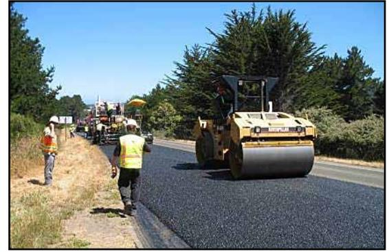
Figure 2. Breakdown compaction on Route 1
