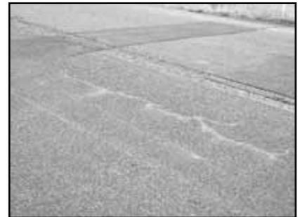
Type of distresses in Route 1. Longitudinal cracking, above, and chip seal raveling, below.
