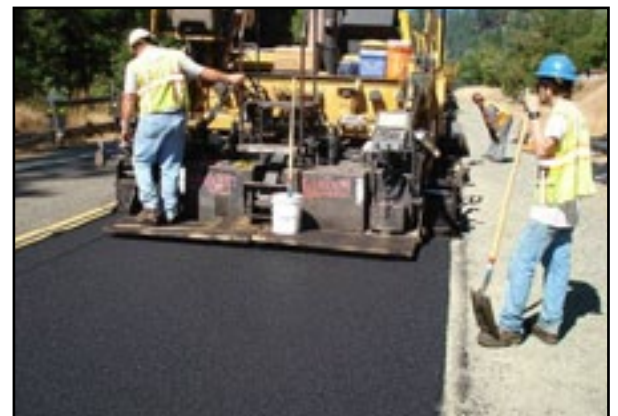
Figure 3. Mix coming out of paving machine after AR2000 recycling train.
