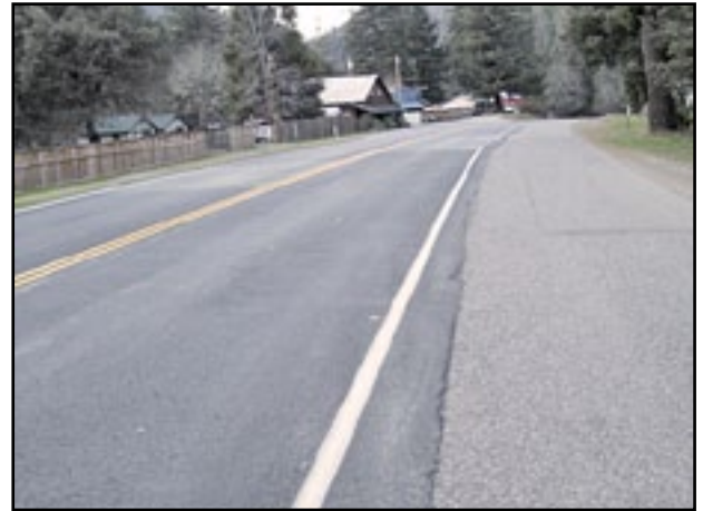
Figure 5. HIR pavement condition after one rainy season and some grinding for improving smoothness
