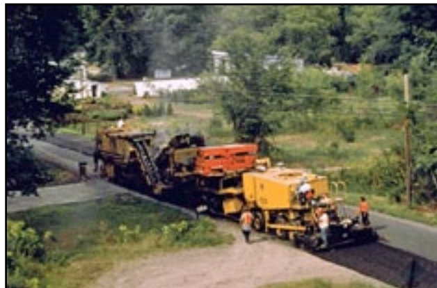
Full depth reclamation. Photo FHWA
