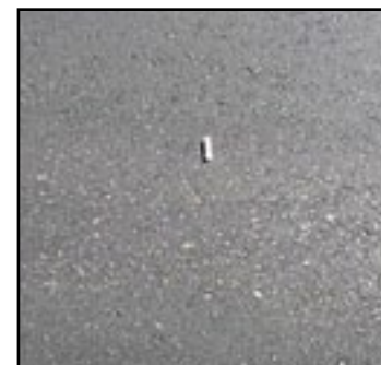
Finished mat with Sasobit
