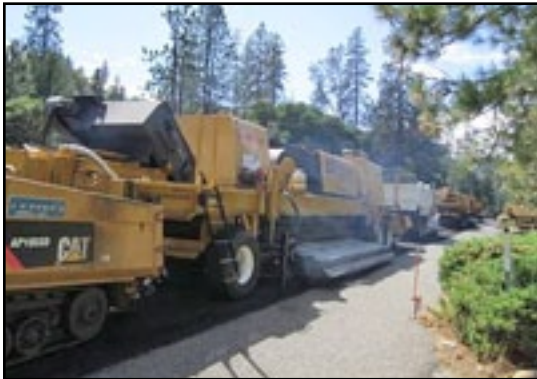
Figure 1. AR2000 hot in-place recycling train in SR 299 Big Bar area.
