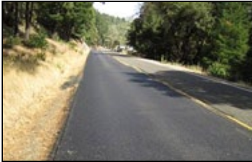
Figure 4. Finished HIR section alongside of existing old pavement.
