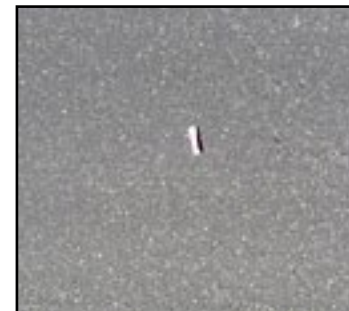
Finished mat with no warm mix additive
