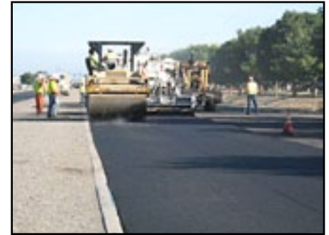
Paving with PG76-22TR
