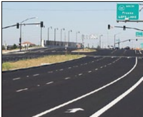
A microsurfaced treatment in Elk Grove, California.
