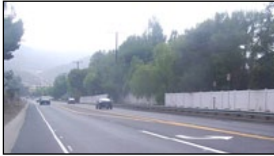
Left, construction on Kanan Road; and above, the completed project,
