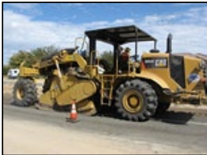
Figure 4. Mixer/reclaimer used for FDR
