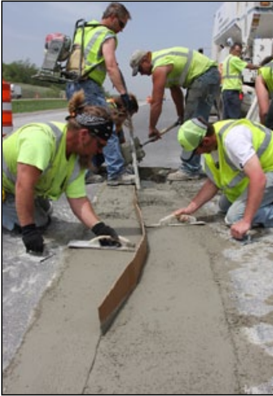
Fig. 2. PDR concrete placement operation.
