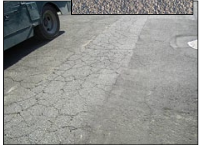
Figure 4 (below). Double chip seal after five months of service.
