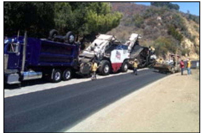
Construction of Encinal Canyon Road
