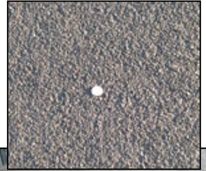
Figure 4 (below). Double chip seal after five months of service.
