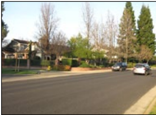
Figure 2. Completed project in City of Roseville.
