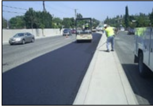
Construction of Halliburton Road at Stimson Ave.
