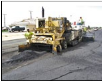
Figure 3. Paving the recycled mix
