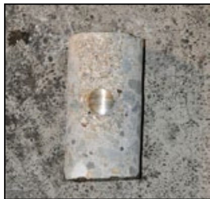
Figure 5. Core showing improved consolidation with the polyester polymer grout.
