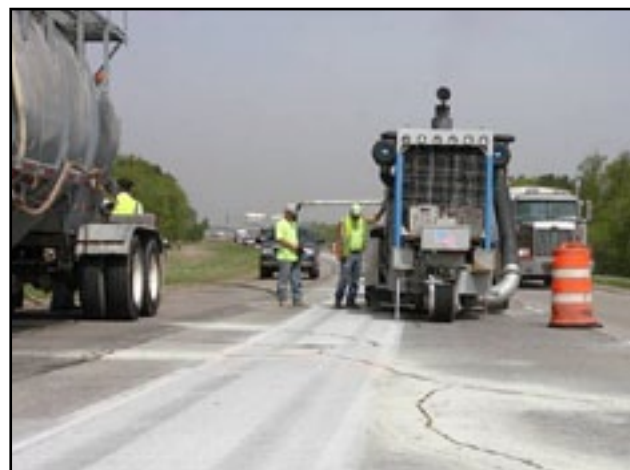
Fig. 1. Completed PDR prior to diamond grinding.
