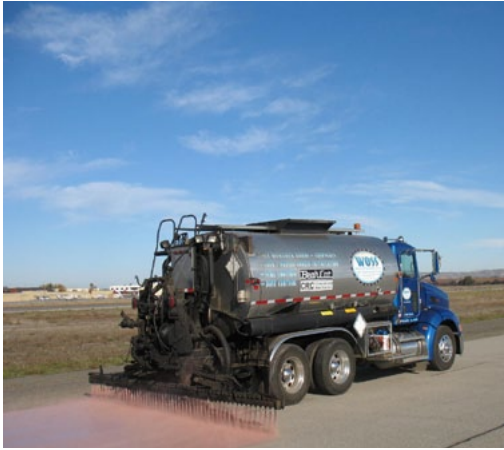
Application of Reclamite Rejuvenator
