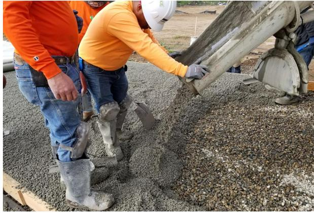
Figure 3. Pouring pervious concrete over drainrock base
