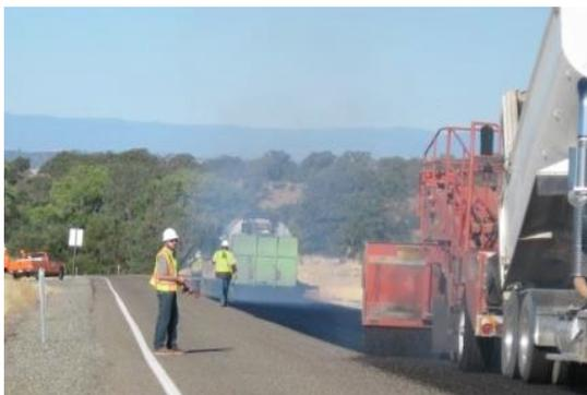
Figure 1. Typical AR Chip Seal Construction
