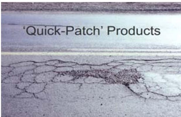
**Pothole filled with quick-patch material**
