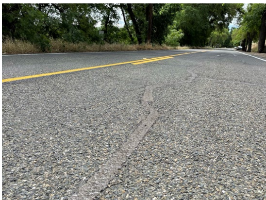
Composite Seal On Asphalt Pavement (Hwy 160 Sacramento)
