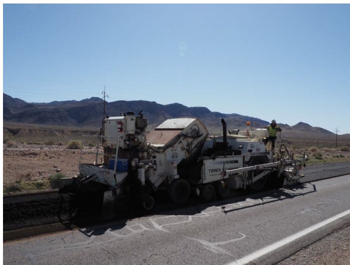
Paving the CIR mixture
