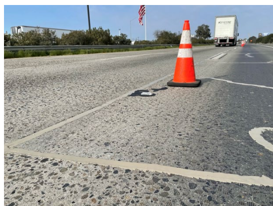
Composite Seal On PCC Pavement (Hwy 99 in Fresno)
