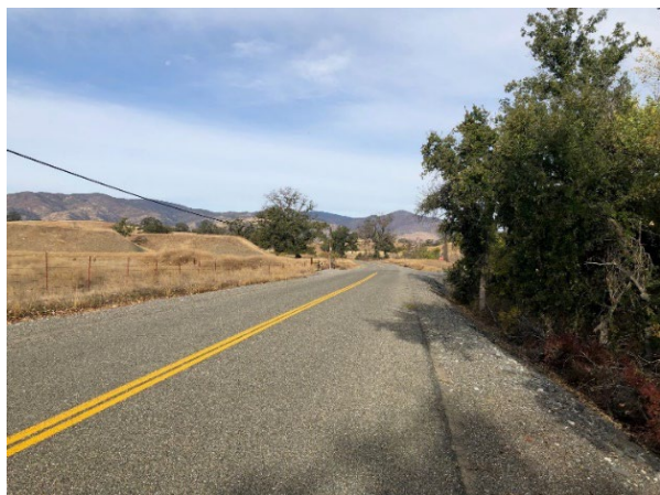
Figure 6a. First chip seal applied (overview)
