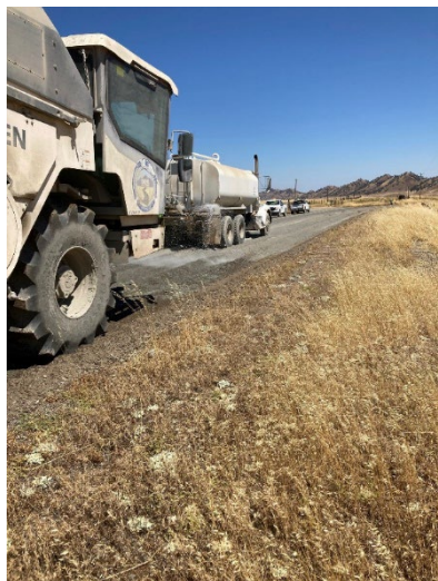
Figure 2. Adding water to the cement and mixing
