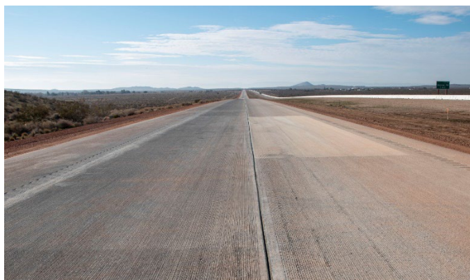
The completed southbound CRCP lanes – ground and grooved.
