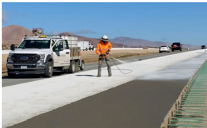
Spraying curing compound onto the fresh concrete. Photo courtesy of Caltrans.
