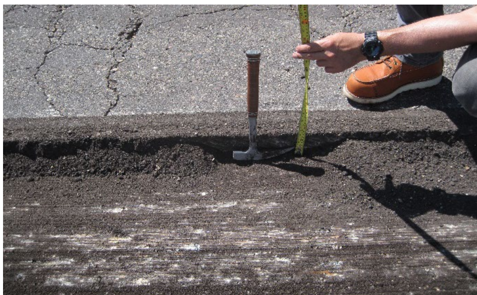
Checking recycling depth using a Rock Pick on a PDR project.
