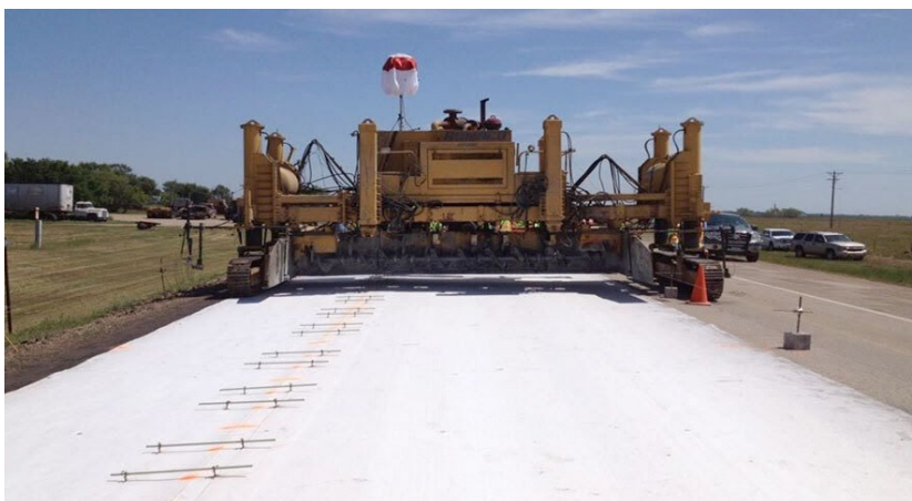
Concrete overlay being placed (Source: Jerry Voigt)
