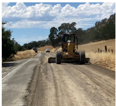
Figure 3. Finishing the grade
