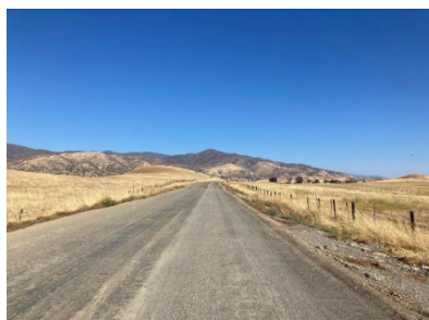
Figure 4. Fog sealed surface
