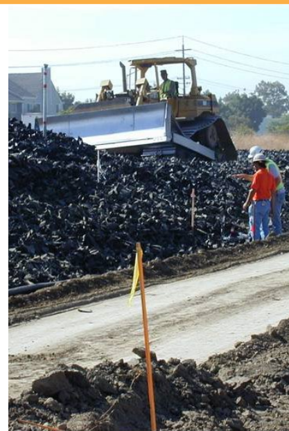
Dixon Landing Embankment Completed
