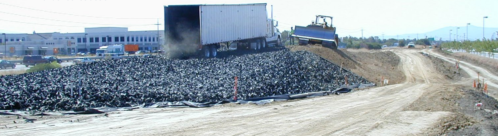
Dixon Landing Embankment Fill under construction
